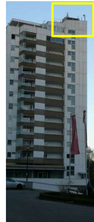
02 DEC 2016 Mobile phone base station No. 240224 at Im Druseltal 12: installation height 37–40 m (121–131 ft), 9 sector antennas
