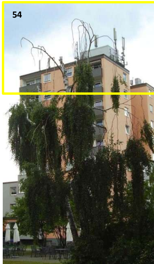
08 JUL 2008 Mobile phone base station at Hauptsmoorstraße 26 a, courtyard. Birch tree (view from the northeast)
