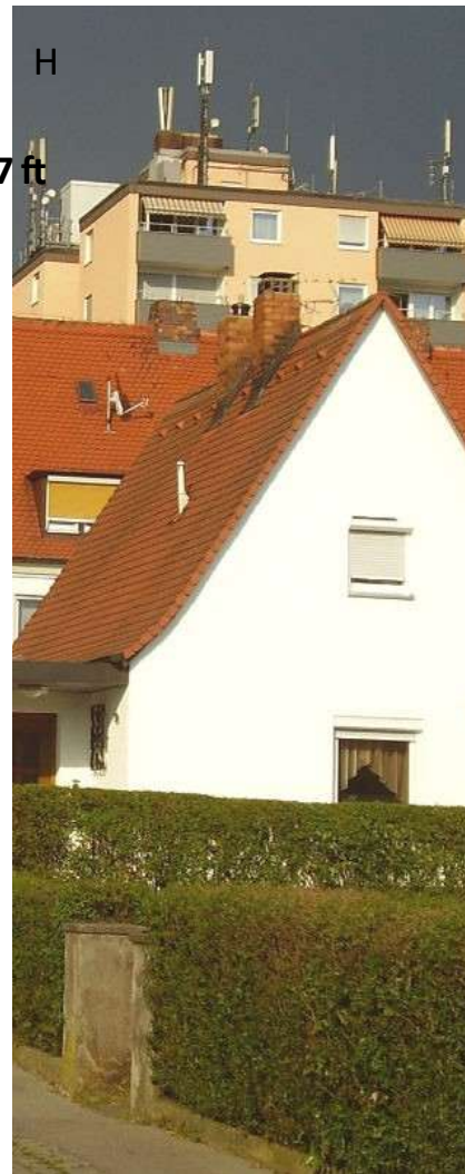
Mobile phone base station at Hauptsmoorstraße 26 a
