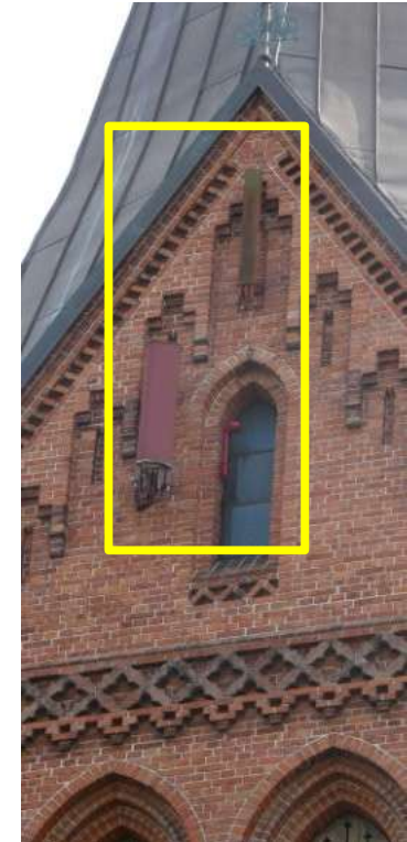
Section of the north side of the church steeple with antennas, which are painted red. According to the site certificate, there are eighteen 330° antennas that radiate toward the spa gardens.
