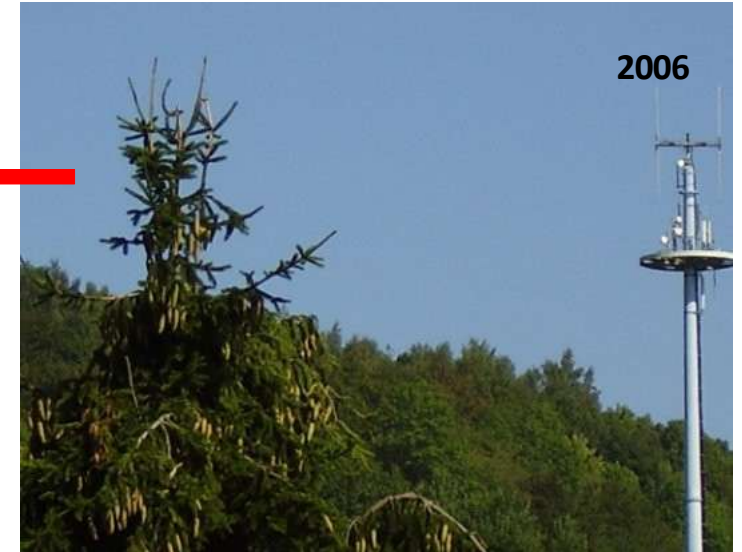
Mobile phone base station No. 890015, above Steinbach-Hallenberg
