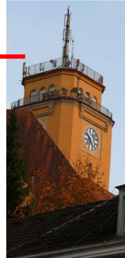
01 NOV 2014 Mobile phone base station at the Markgraf Ludwig High School. Four 260° antennas reach the trees along the Lichtenthaler Allee.
