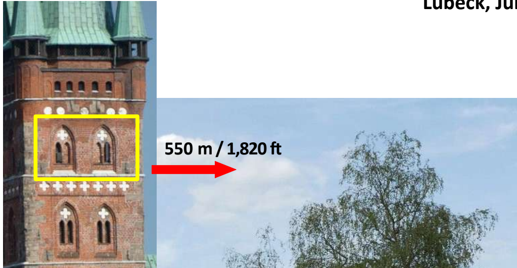
St. Peter's Church, south side of the tower with mobile phone base station antennas
