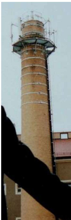
A mobile phone base station is mounted at the courthouse chimney.
