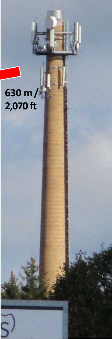
Mobile phone base station at Ottelmannshäuser Str. 3
